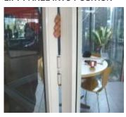
Lift the panel up and into position. Try to keep the panel as vertical as possible.
