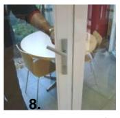
Close the active panel (panel with door handle). Lift handle upwards (indicated in picture) to draw the active panel hard up against the seals.
