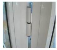
Lower the panel, making sure that the hole in the hinge knuckles have threaded onto pins.
